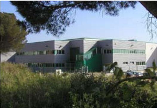
The Procap plant in Llagostera
